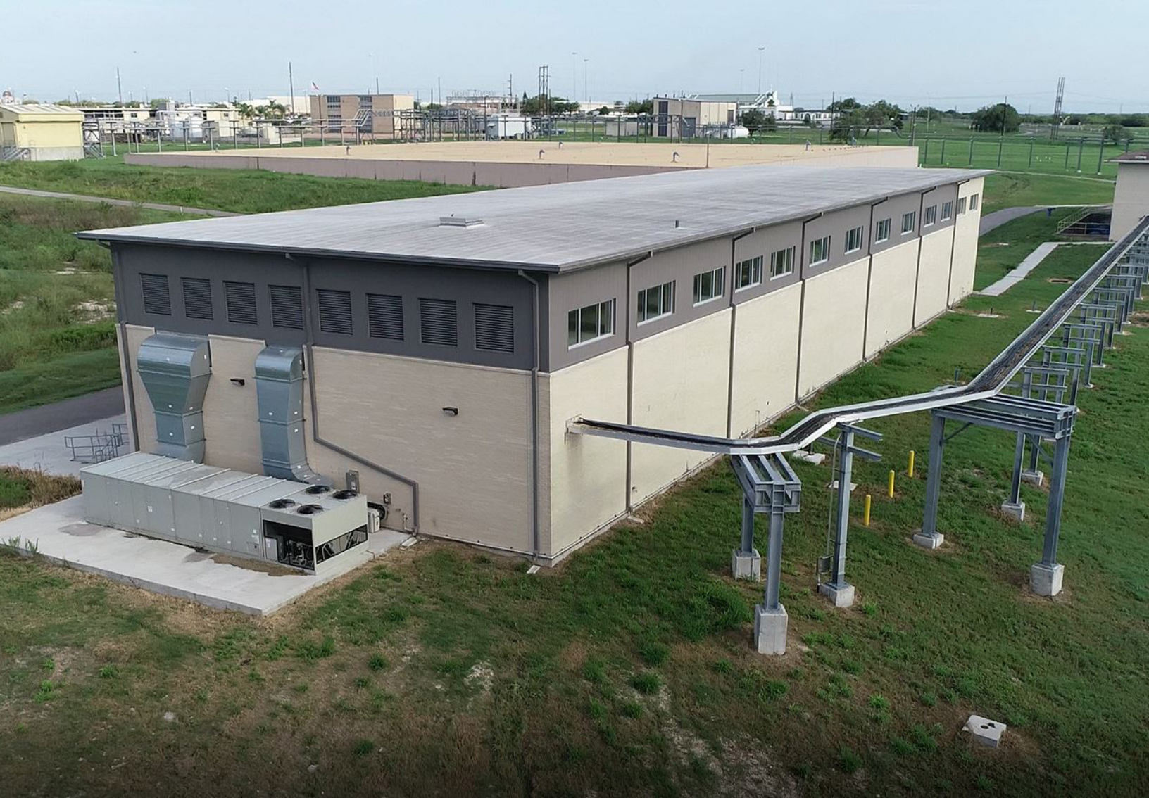
High Service Building No. 3 | O.N. Stevens Water Treatment Plant | City of Corpus Christi, Texas
